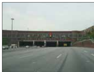
Reconstruction of the old Elbe tunnel tubes (A 7)
